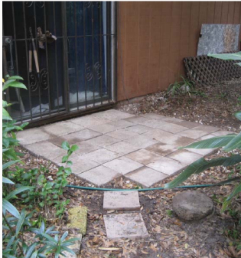
Here the blocks are laid back down
