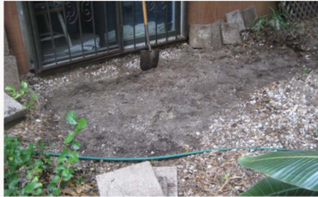
It only took 45 minutes to dig up the old blocks.
