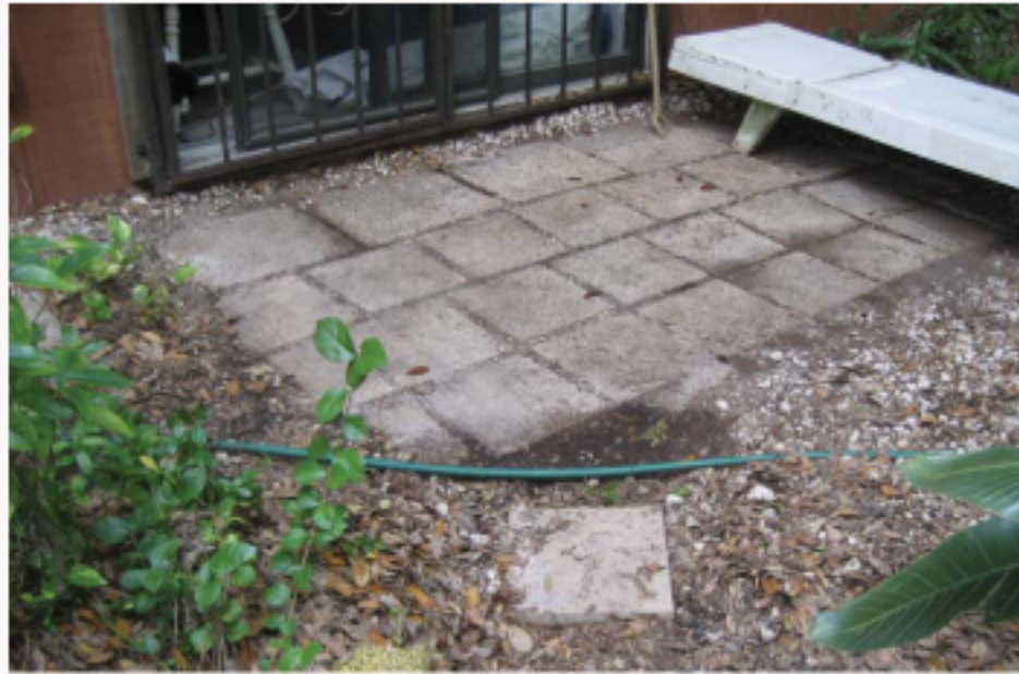
The original patio circa 1997, newly found under layers of dirt and gravel.
